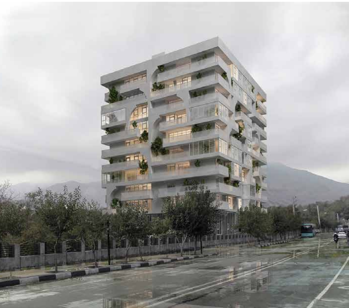
Siddah Chenar Mansion
